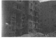
reconstruction of Jad building Saïda, July 20th 1982
